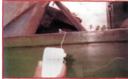
Temperature checks for the mix
