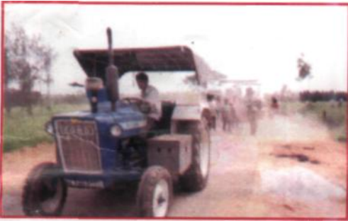
Surface cleaning using air compressor
