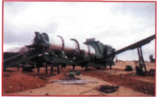
Erection of Hot Mix Point
