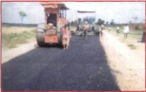
SDBC in progress
