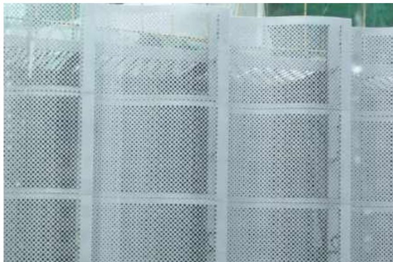
Perforated metal panel, for the concourse elevation in the merging Loop option
