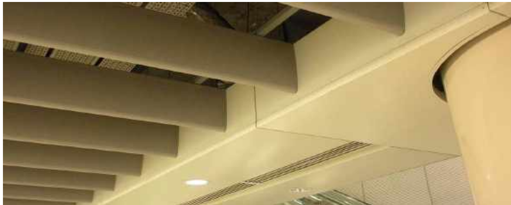
Acoustic panels with open joints to allow leakage point to be identified, if any above - recommended for the Concourse area.
