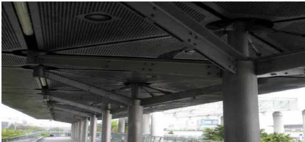
Perforated metal panel are proposed to be used for the finishes of the inner face of the platform roof.
