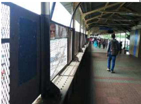
Existing FOB of Bengaluru City Station(SBC)
