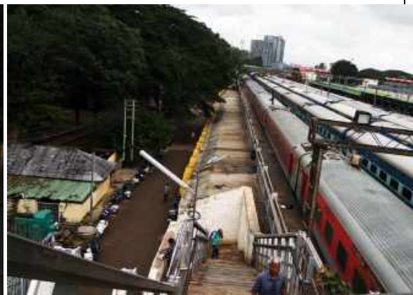
Back side of the SBC Station showing staircase connectivity with FOB
