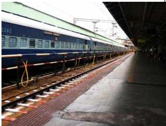
Existing Platform of Bengaluru City Station(SBC)
