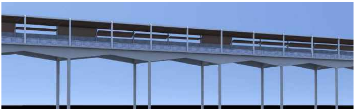
North elevation of FOB from Track yard level
