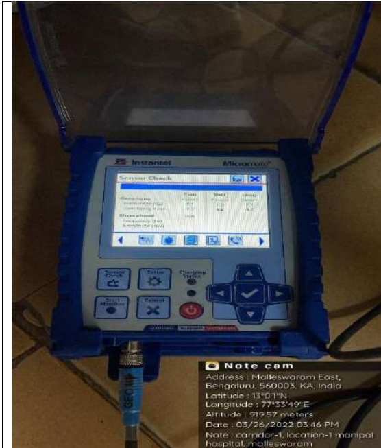
Corridor-1 V-1, Manipal Hospital, Malleshwaram
