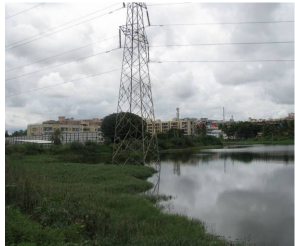
Picture 2b: One of the two electric towers erected on the lake.
