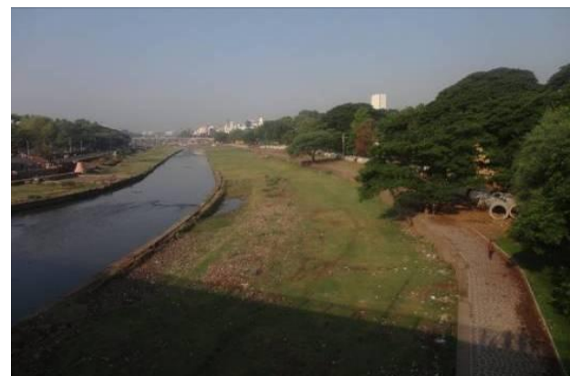
Plate 6-3: River Improvement works under JNNURM
