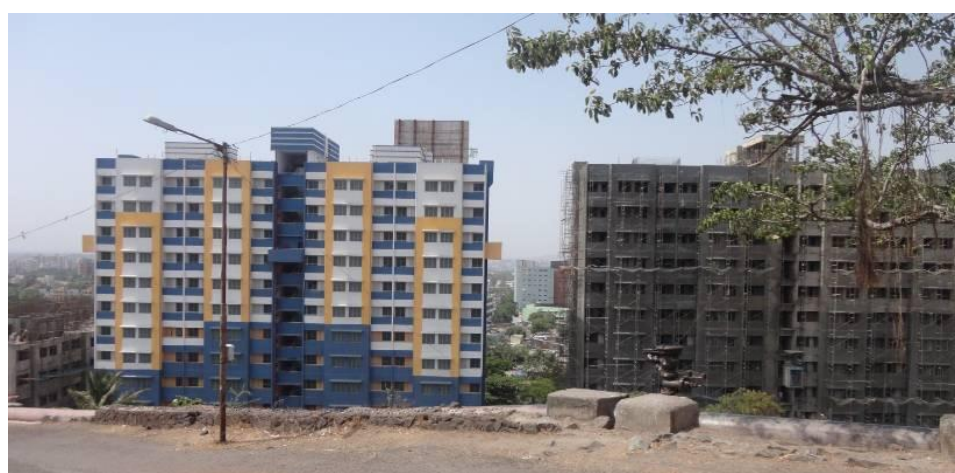
Plate 3-10: Housing for slums under construction at Hadapsar
