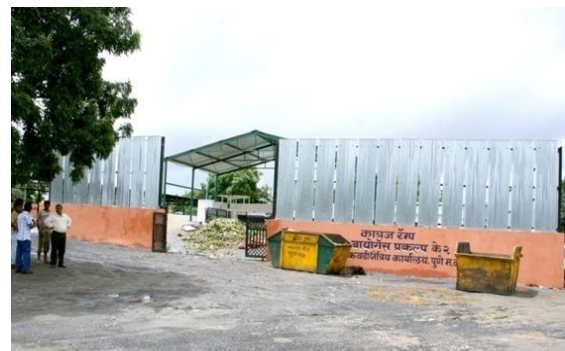
Plate 4-6: Katraj Bi-gas Plant
