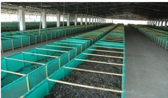
Plate 4-5: Disha Waste Management Plant
