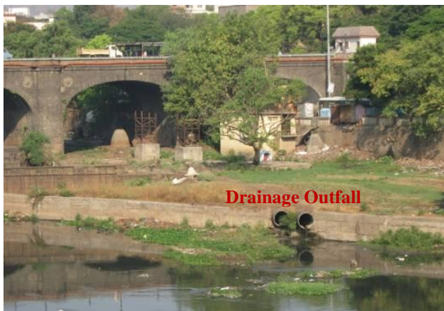
Plate 6-4: Drainage outfall into the river
