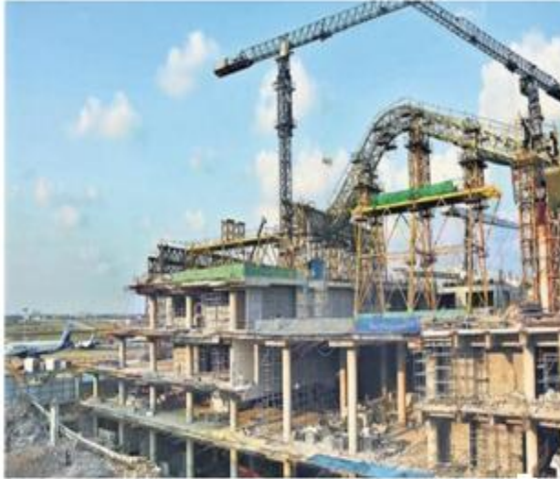
Construction activites in Chennai International Air port
