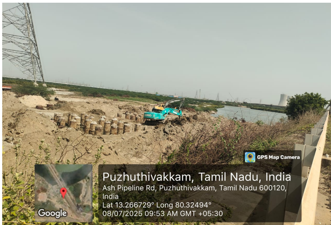
Figure 11: Ongoing works to remove concrete structures located on land and along the riverbanks, but not from within the river. Photo dated 08 July 2025
