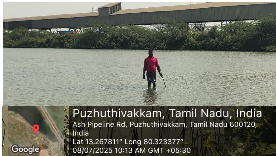
Figure 12: Depicts below-knee level depth at the concrete structures removal site-Konamudduku. The construction debris and sand have settled in the river bed decreasing the depth in this region. During low tide, boats are unable to pass through this region. No efforts have been made to remove the foreign materials from the river bed.
