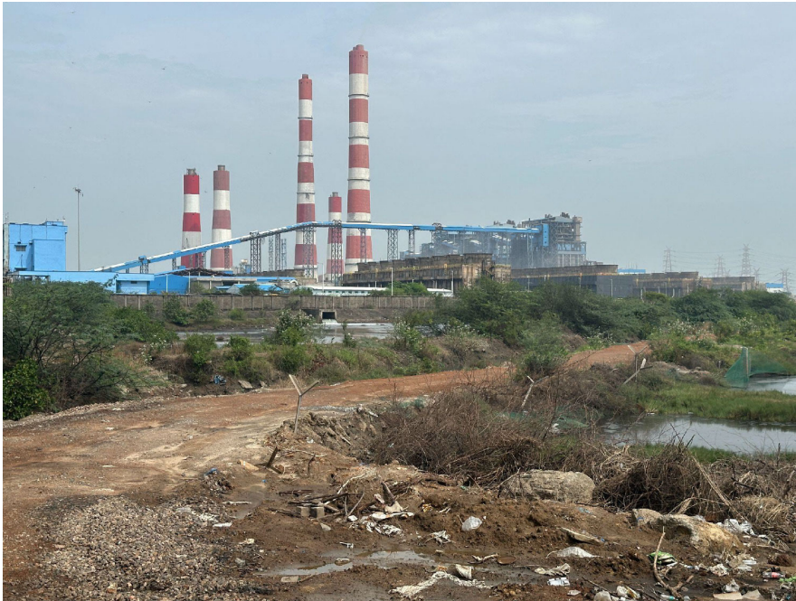
Figure 2: Hot water discharge outfall from NTECL
