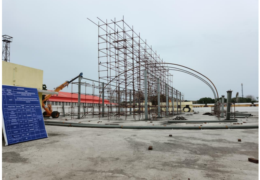
Figure 13- Ennore bus depot under construction
