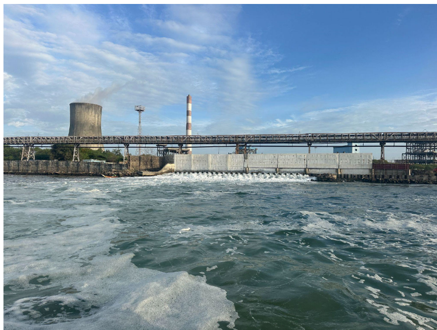
Fig. 1 Hot water discharge into estuary from NCTPS
