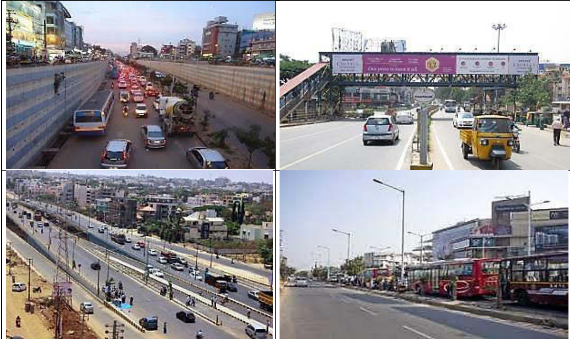
Figure 2- 2: Photos of Outer Ring Road along the proposed corridor
