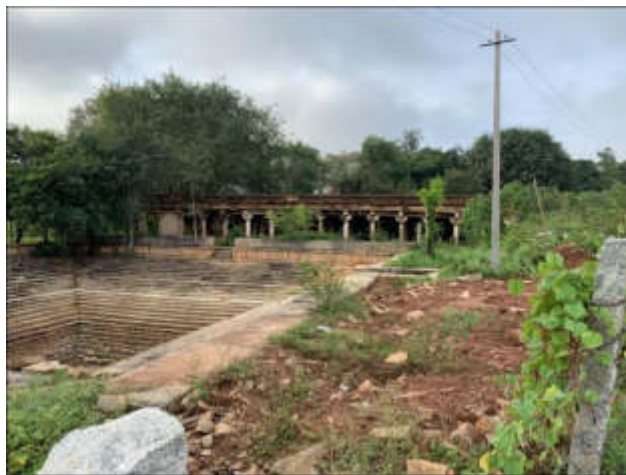
Figure 11: Most vibration sensitive structure in the project area – Chikkajala Old Fort and Temple @26+574km, 26.35m away, phase 2b
