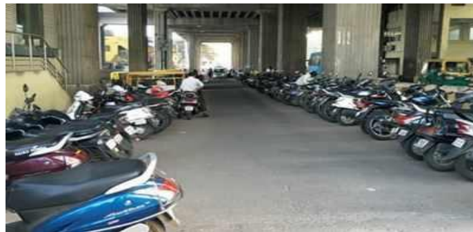
Figure 15.10 Detection of unauthorized/illegal Parking
