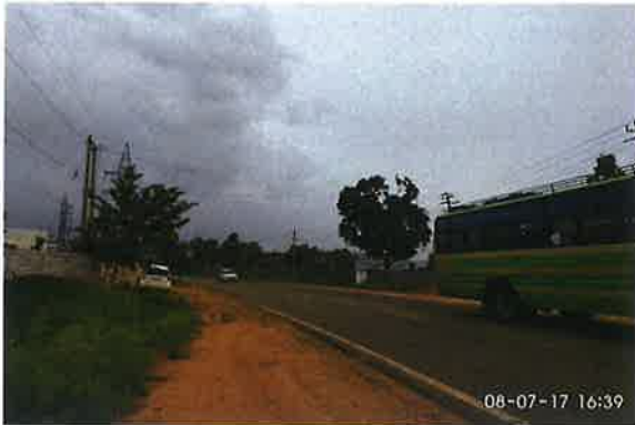
Project Start Road (Km. 0.700)
