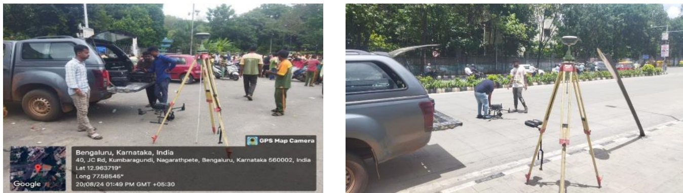
Figure 40: Topography Survey on Site
