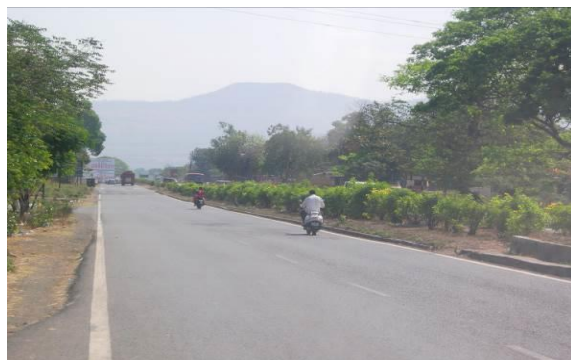
Existing Condition of NH - 04
