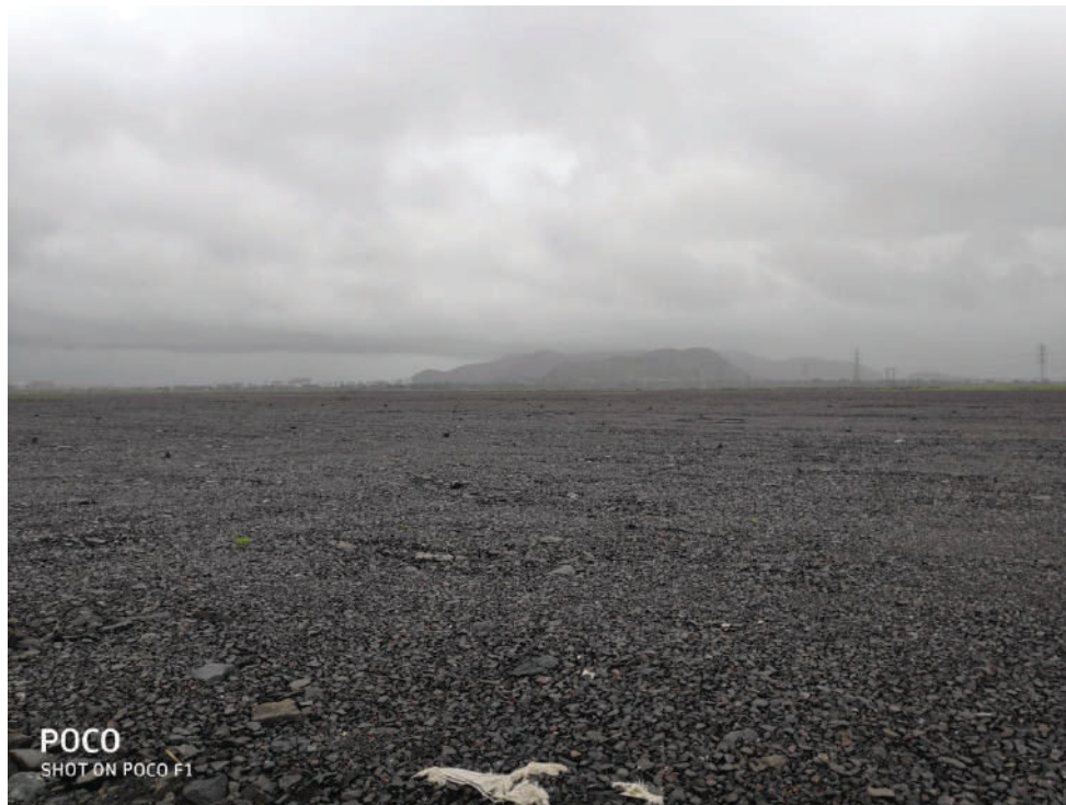
Photo 4 : Reclaimed Ground Level Area of NMIA Filled upto 5.5 m RL.
