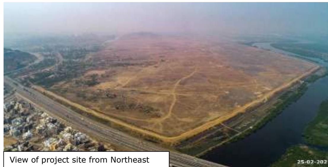
FIGURE-1.2(D): PHOTOGRAPHS SHOWING WORK COMPLETION STATUS OF PROJECT SITE
