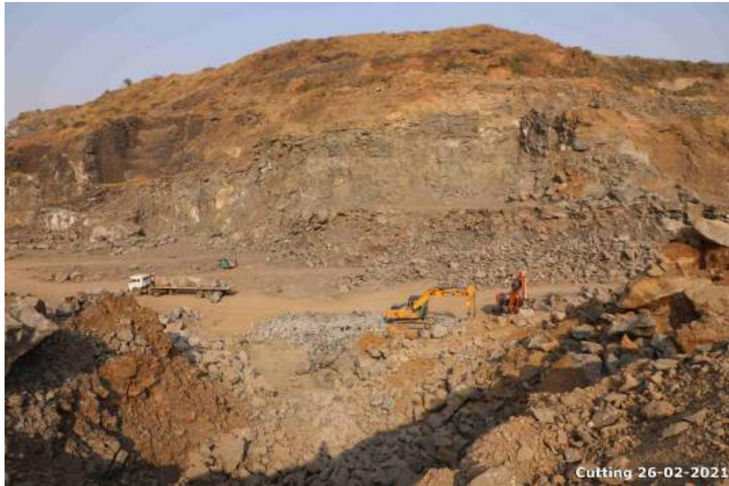
FIGURE-1.2 (A): CUTTING OF ULWE HILL AT PROJECT SITE
