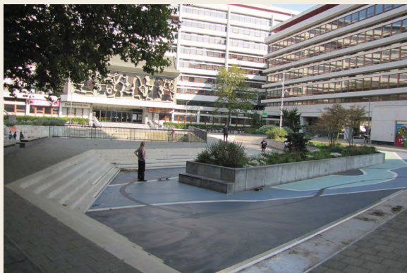
Benthienheim Water Square in Rotterdam, an example of integrated multi-use blue-green-grey solution, a conventional play and sports areas with permeable surface that doubles as an unconventional stormwater catch basin.
