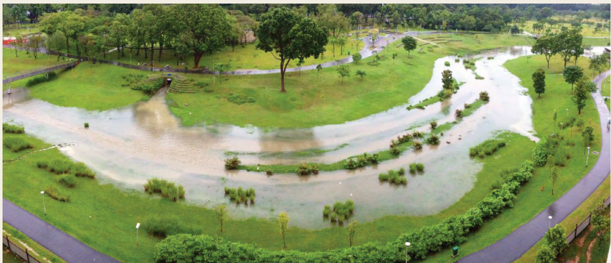
The Bishan-Ang Mo Kio Park, Singapore uses blue-green infrastructure for flood control, biodiversity management, microclimate control and adds a high-quality public space asset to the city for recreation and educational use.
