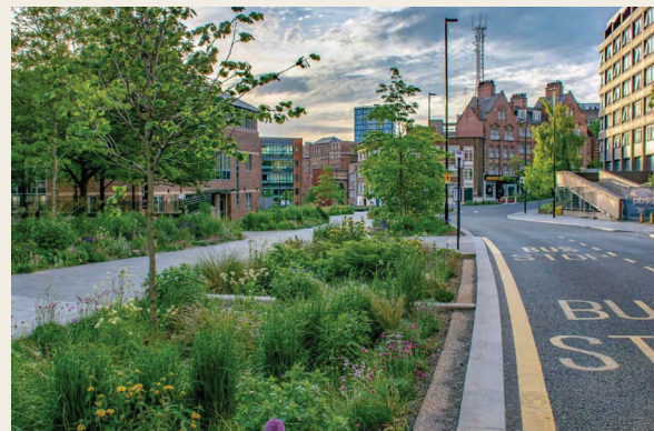
Green street section in Sheffield with permeable lane surfaces, planters, and rain gardens to enable stormwater management.
