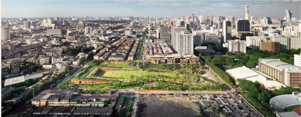
An 11-acre rooftop park in Bangkok's commercial district directs runoff into a retention system reducing pressure on underground drainage and sewer systems.
