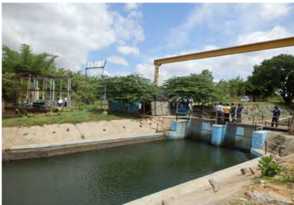
Photo 3.2.1 Gate for Canal Intake
