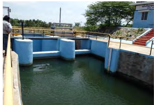
Photo 3.2.2 Gate for Pipe Intake
