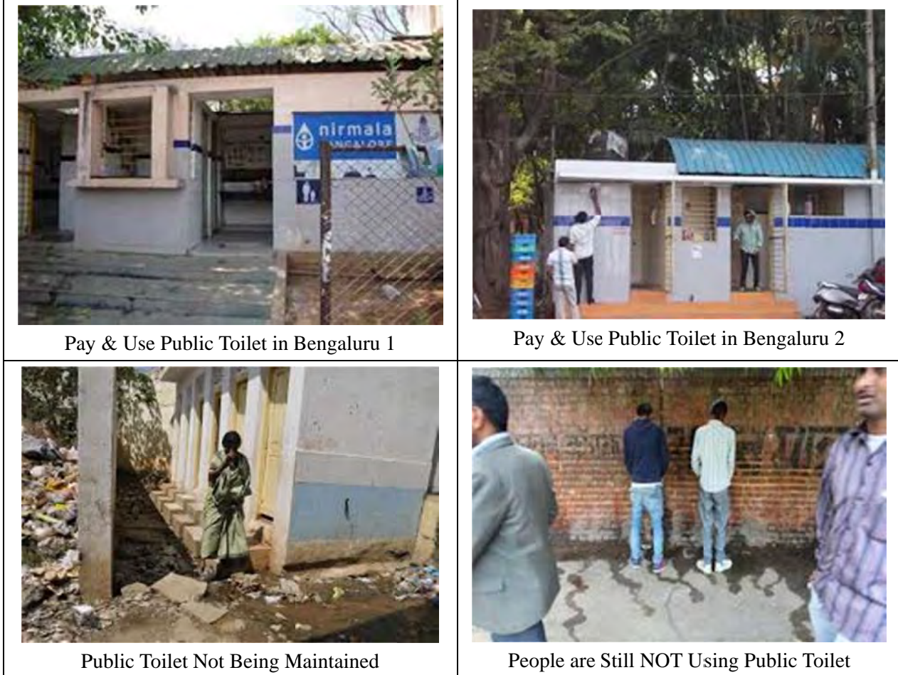
Photo 11.2 Actual Conditions on the Existing Public Toilet in BBMP Area
