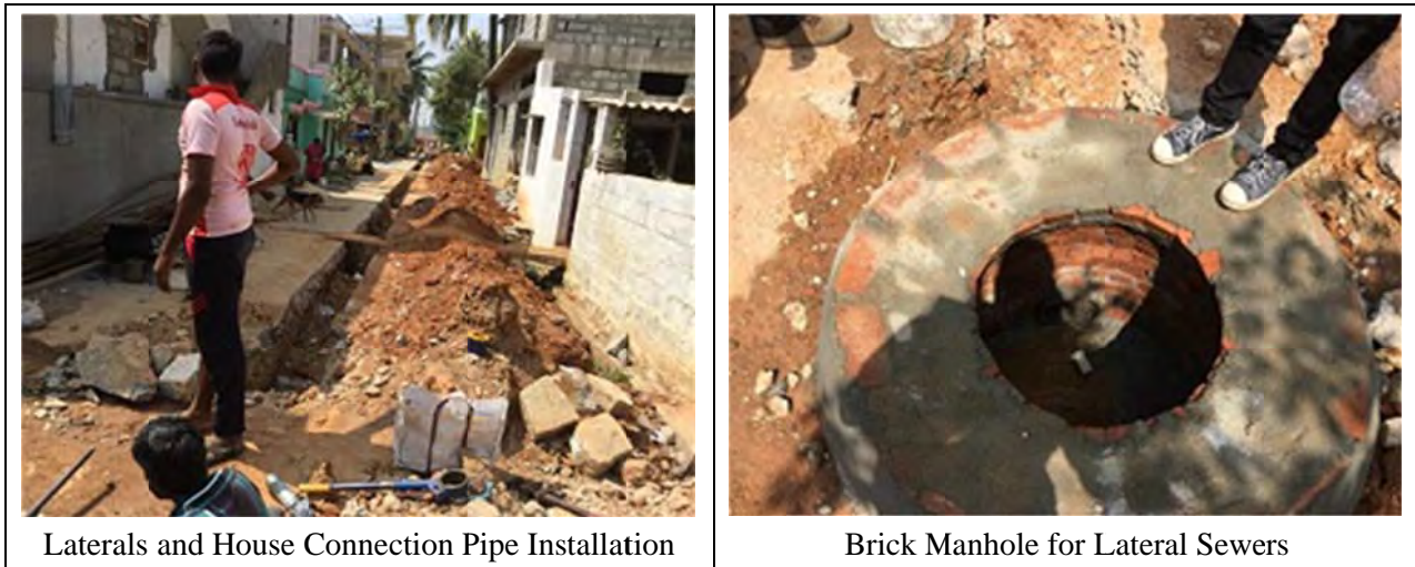
Photo 11.1 Actual Construction Site of Lateral Sewers and House Connections
