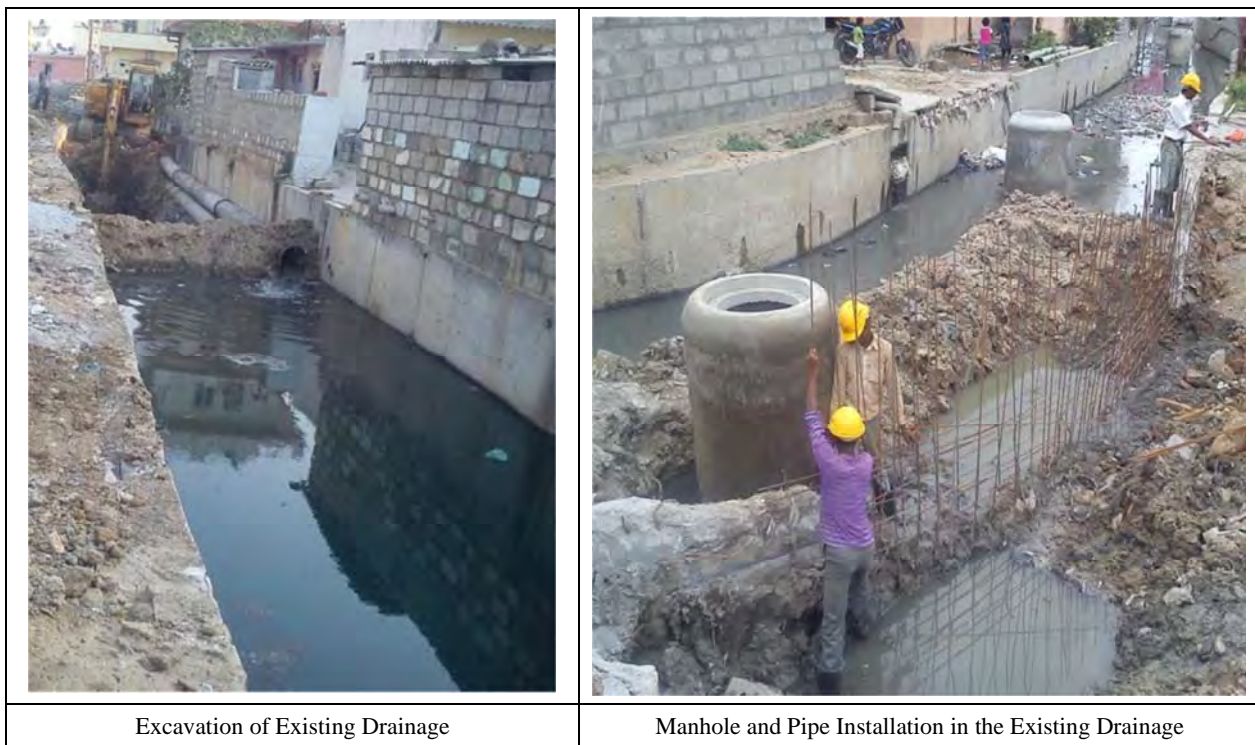
Photo 10.2.21 Installation of Sewer Line under Drainage Bed
