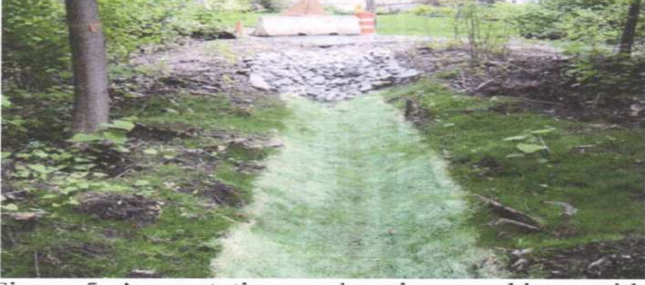
Figure 5. A vegetative swale using a sod base with a rock filter at the end of the swale.
