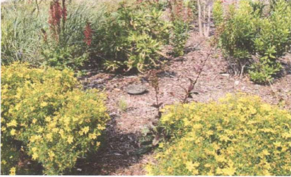
Figure 4. An infiltration basin/bed utilizing vegetation to make the structure looks more aesthetically pleasing.
