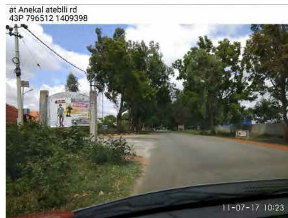
Road Site Plantation along the Road (Km Ch. 140.93)
