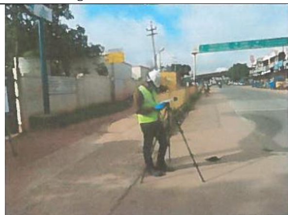
Ch. Km 9.200 at NH-48 (NH-4) near to Junction of Dabaspete
