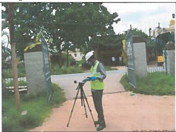
Ch. Km 30.700 at NH-75 (NH-48) near to the Junction of Gudemaranahalli
