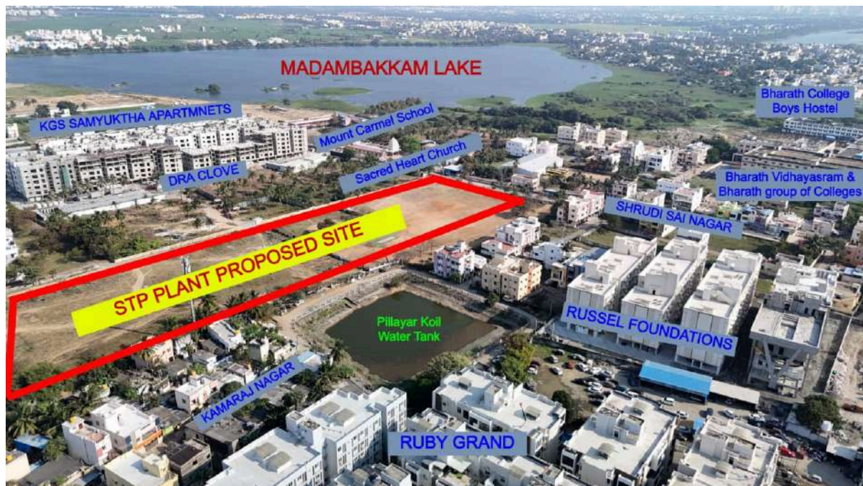
IMAGE SHOWING THE PROPOSED SITE FOR STP - SEWAGE TREATMENT PLANT AND THE
