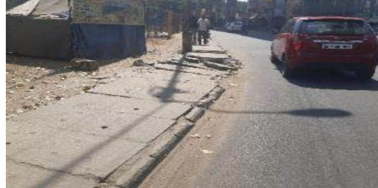
Figure 97 Damaged footpaths slabs
