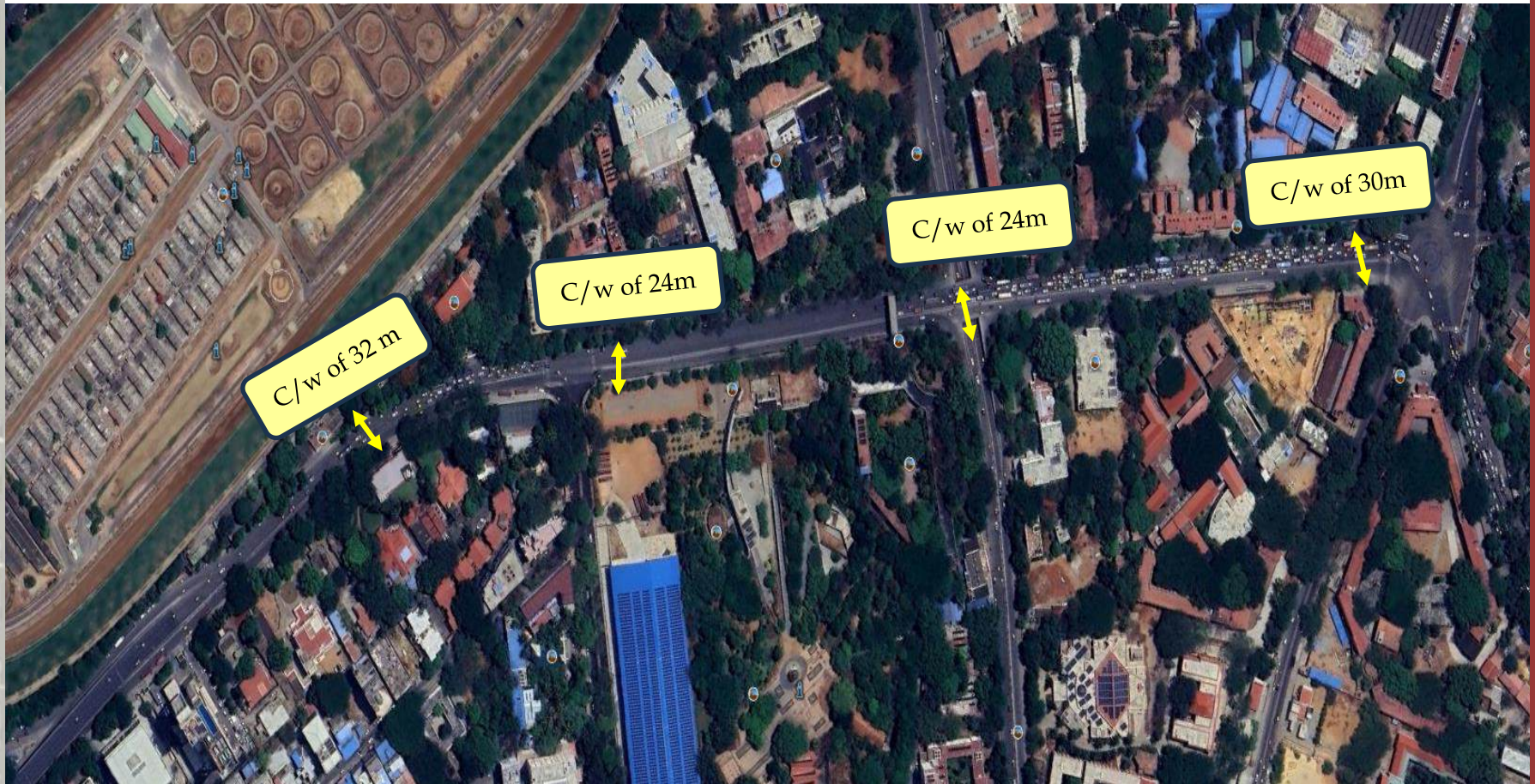
Figure 246. Road inventory data from Anand Rao Flyover to K.R. Circle
