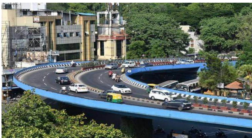
Figure 44. Turning Radius at Yeshwanthpur Flyover
