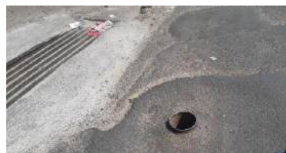
Water Valve is projected out dangerously
