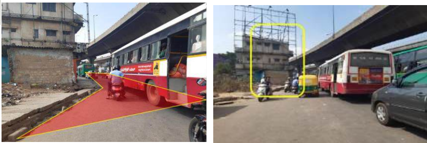
Figure 72. Issues at SRS Junction.
