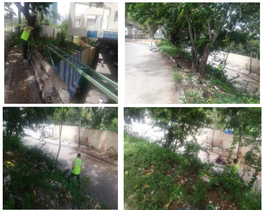
Figure 54. Measurement of Steep Slope at Mysore Sandal Soap Factory
