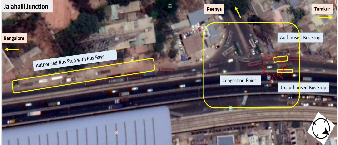
Figure 74. Issues at Jalahalli Junction.
