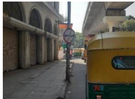
Sign Board not as per IRC near Trinity Circle
