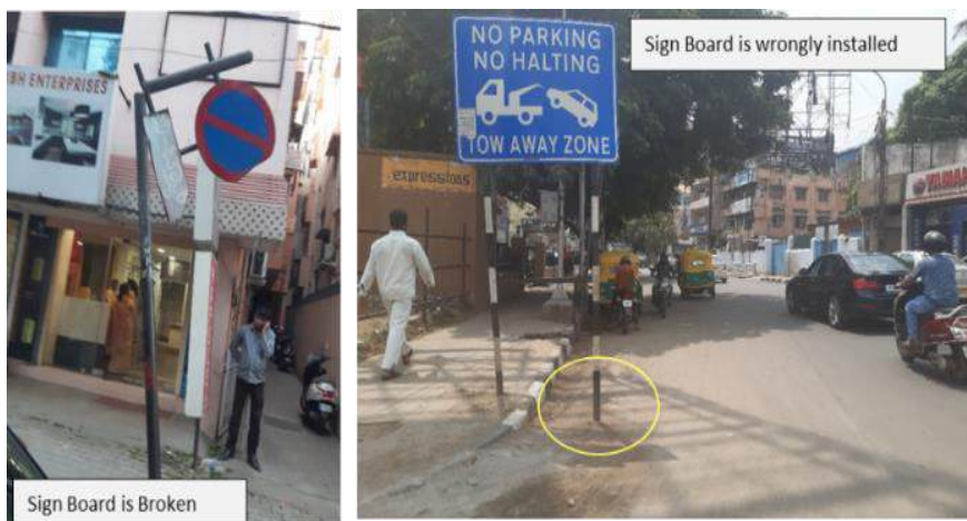
Figure 148 Dislocation of Signboards Along The Corridor
