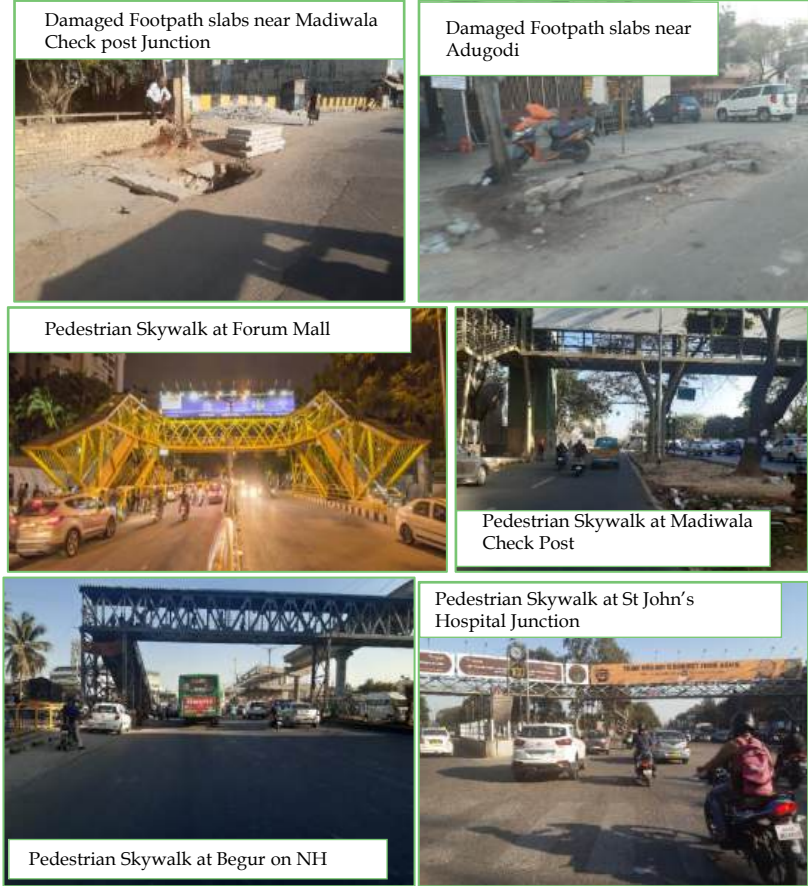
Figure 257. Absence of Pedestrian accessibility to Metro Stations from LHS
