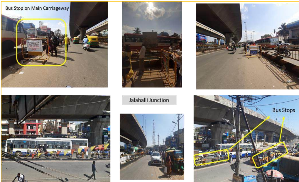
Figure 75. Issues at Jalahalli Junction.
