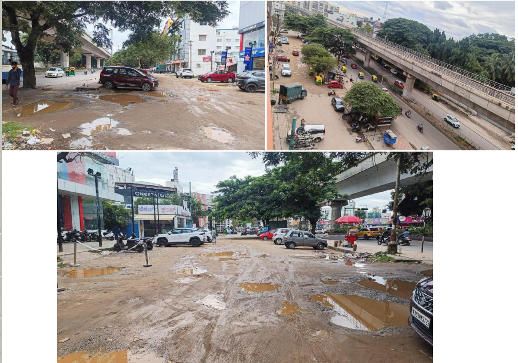
Figure 238. Site inspection Photos
