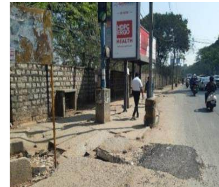
Bus Stop Condition along the corridor
