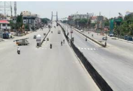
@ K.R.Puram Hanging Bridge
