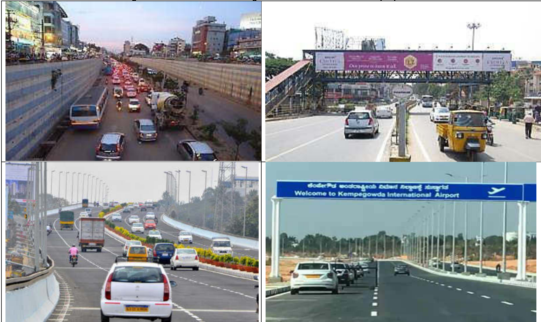
Figure 2- 7: Photos of Outer Ring Road where metro corridor is proposed
