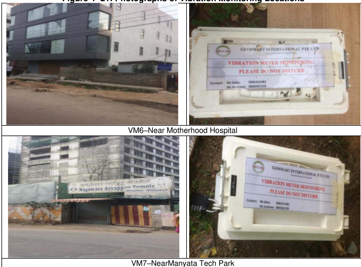
Figure 4- 21: Photographs of Vibration Monitoring Locations
