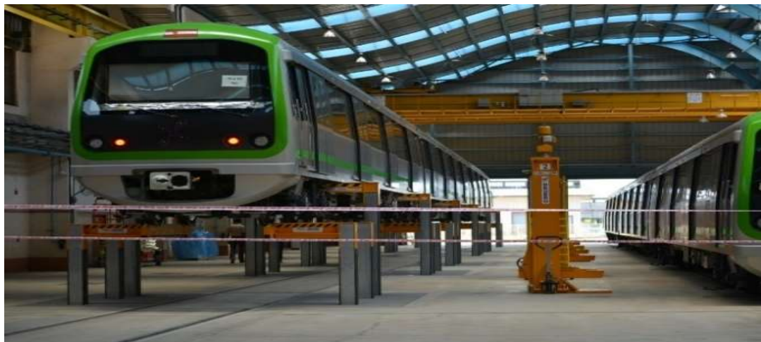
Figure 13.6: View of Work Shop Shed
