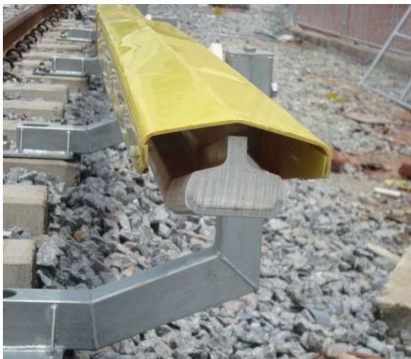
Figure 12.2 Third Rail and Stringer System
