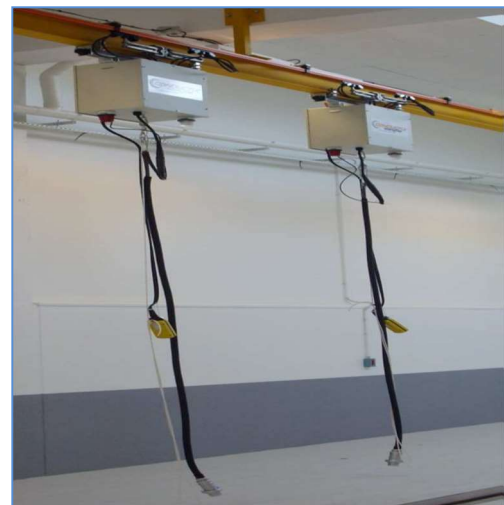
Figure 12.2 Third Rail and Stringer System
