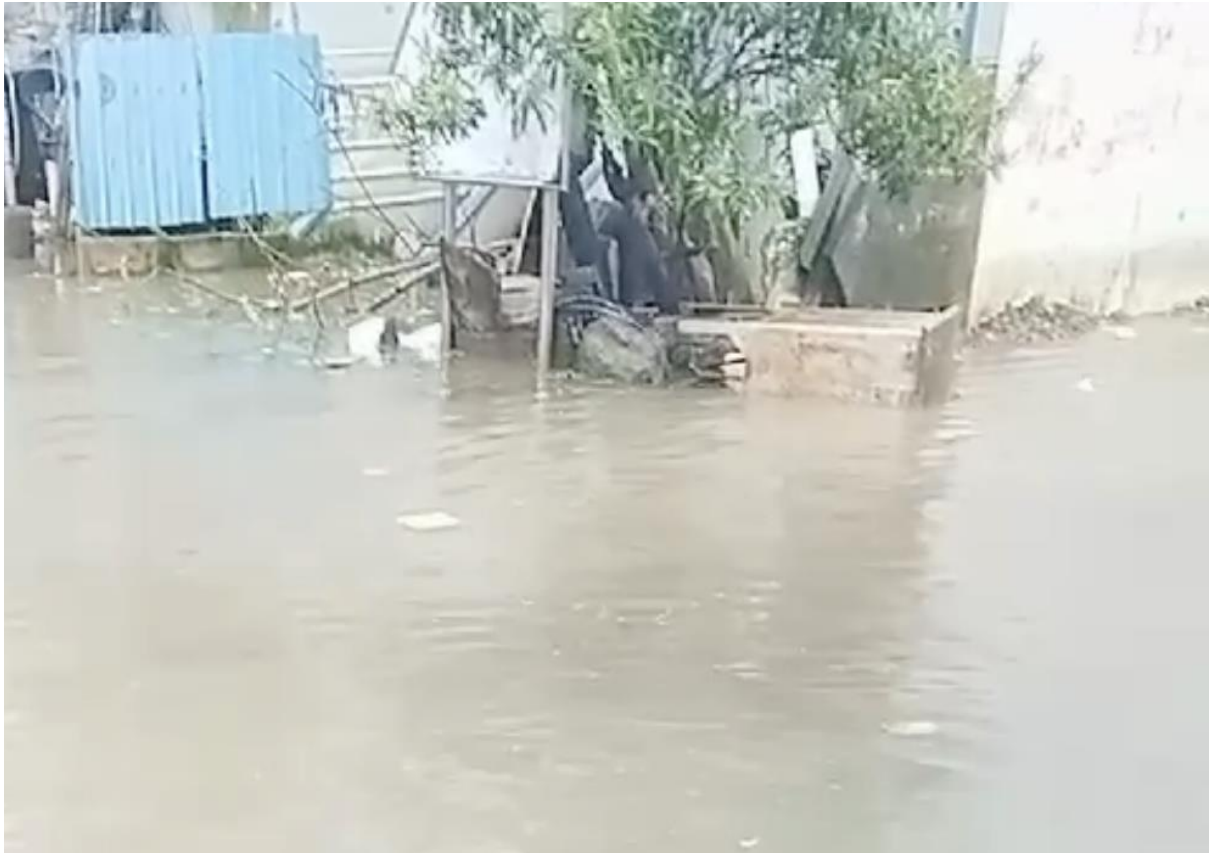
Image 4: Junction box in Semmencherry | Photo: IRCDUC
