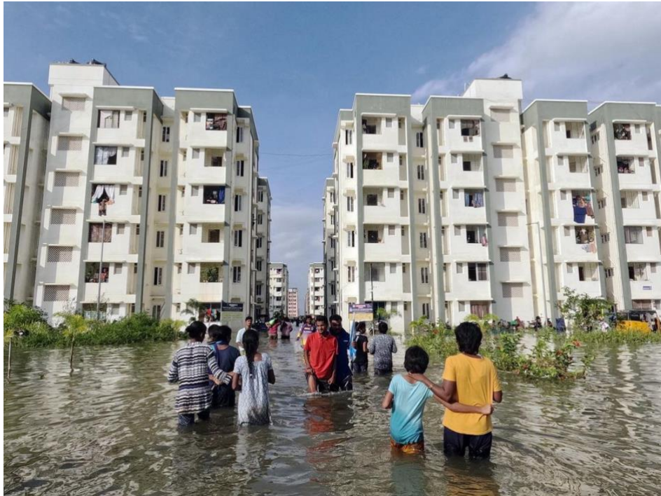
Image 11: Flooding inside the Light House Project | Photo: Palani Kumar
