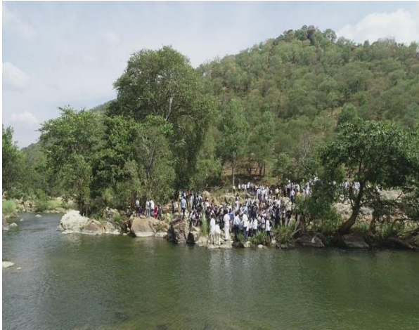
Fig. 1.9: View of Left Flank from River bed along the Dam central line
