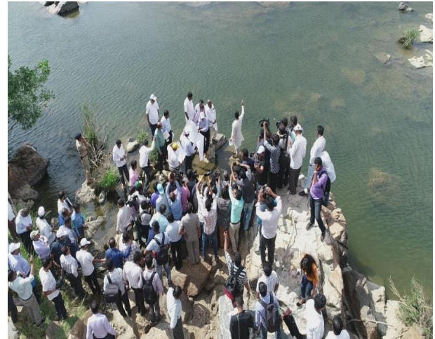
Fig. 1.10: Hon'ble Minister for water resources GOK showing the central line of dam axis
