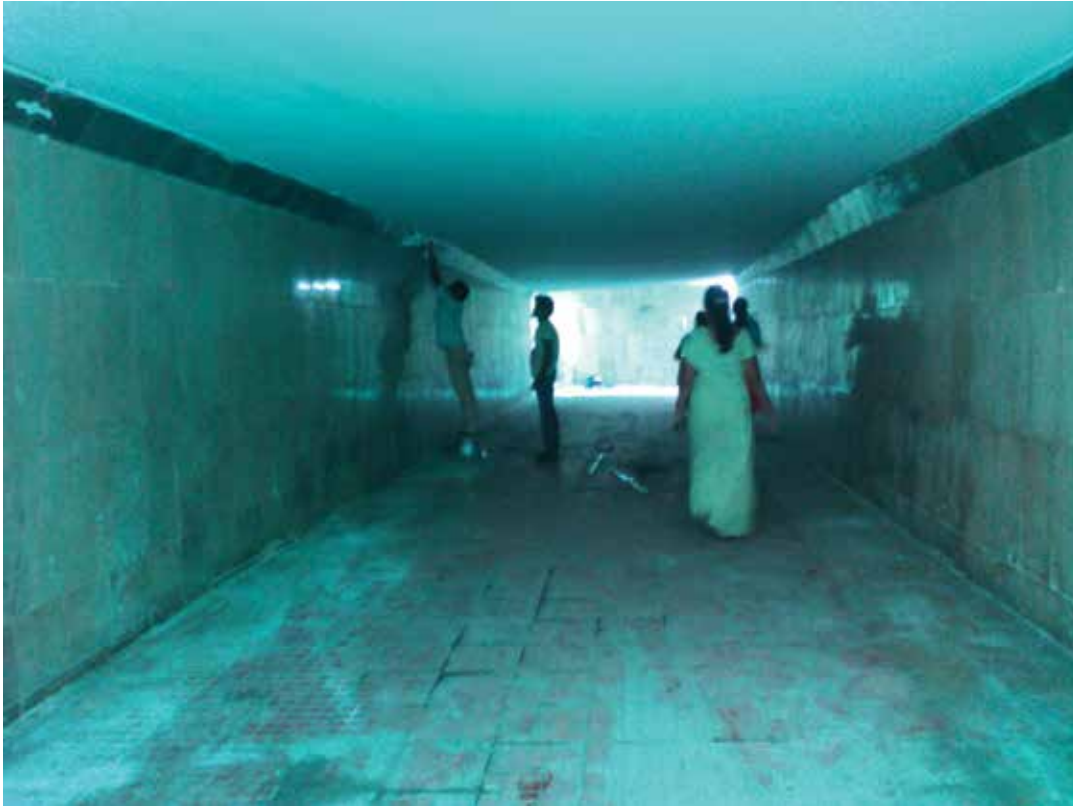
Pedestrian Subway opposite to CDH, T.H Road
