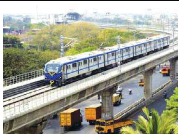
Chennai Metro Rail Limited (CMRL)
