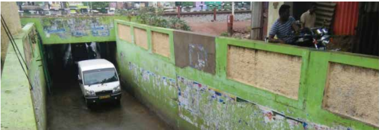
Manickkam Nagar Subway
