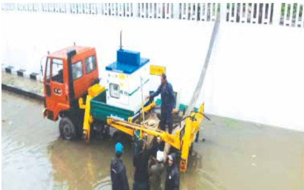
Pump set deployed in subways
