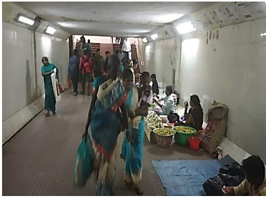
3. Encroachment of Subway
