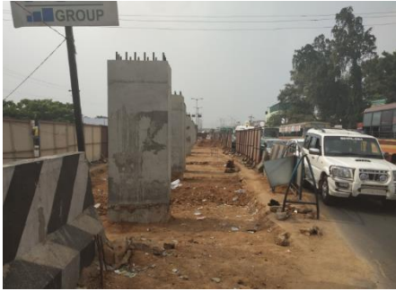
On-going Construction of FOB near the existing Subway
