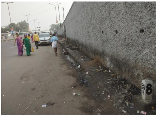
5. Insufficient Footpath & Lack of Maintenance
