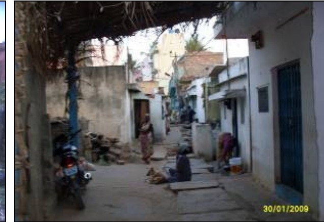
DRAIN NO: BP026 CHAINAGE: 100m. LOCATION: BB Nagara, Kodegehalli Covered drain reaching, providing less scope for drain improvement
