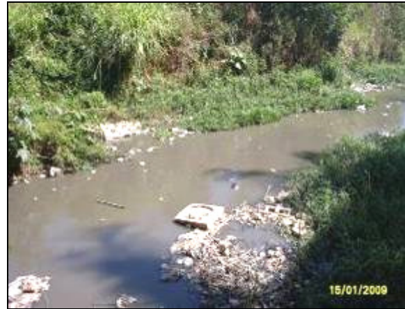
BP183 Ch 550m Waste water stagnation and solid waste accumulation in SWD
