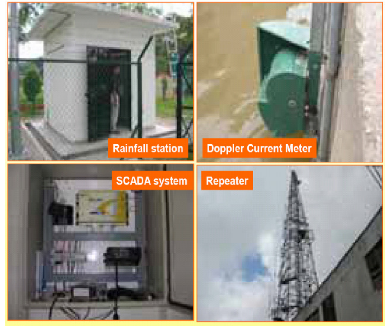
Automated Rain Gauging Station, Current Meter, Data Logger
