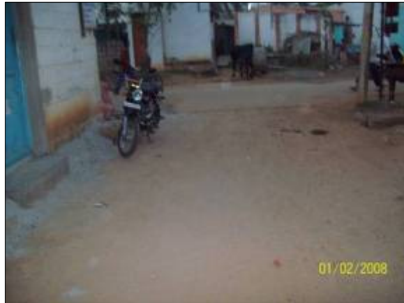
DRAIN NO: RN541 CHAINAGE: 25 m. LOCATION: 3 rd Cross Road to Ring Road, Kengunte Village
