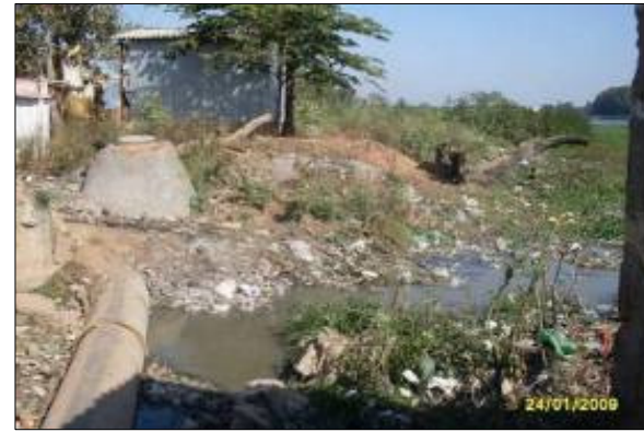
DRAIN NO. BP161 (BY013) CHAINAGE: 1100 M LOCATION :Near Alalsandra Kere Open natural drain with large quantity of garbages/
