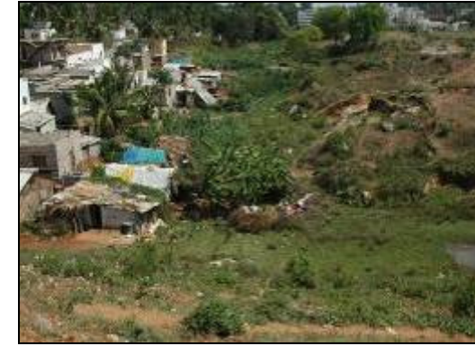
Development of slum area adjacent to SWD near Bandematta area, Kengeri
