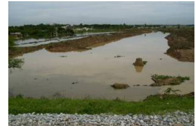
Condition of SWD, at Tannisandra
