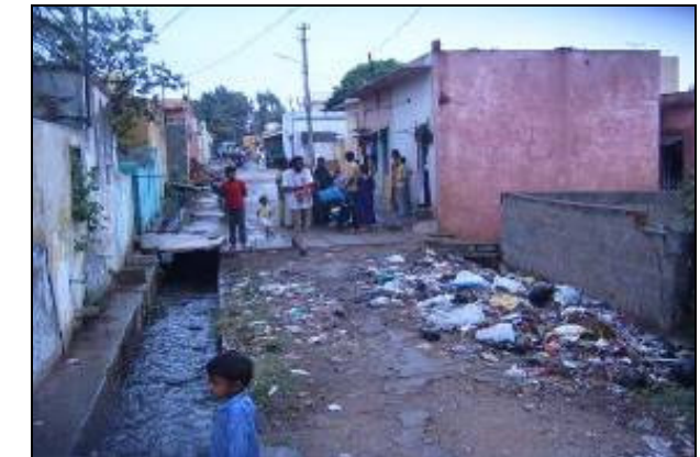
BP155, Ch. 50 m. Srinivasapura layout, near Kogilu Street Sweepings finding its way into SWD
