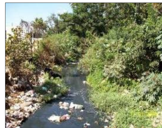
DRAIN NO. DH 213 CHAINAGE :278.0M LOCATION: Vidyanagara Severely silted, large quantity of sewage flow observed
