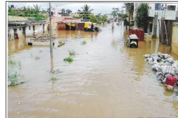
Water surcharged into residential areas at Badarappa Layout, at Hebbal Valley in West Zone
