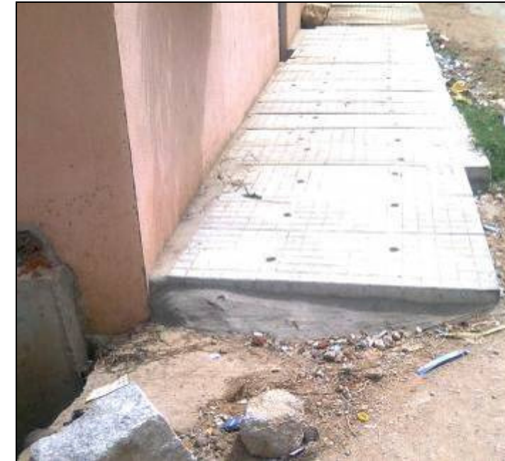
Covering of tertiary / road side drains by pre cast slabs
