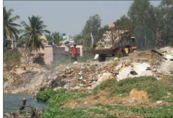
DRAIN NO. MD349 CHAINAGE :3900.0M LOCATION : Marathalli Main Road Large quantity of earth being dumped inside to raise the waterway
