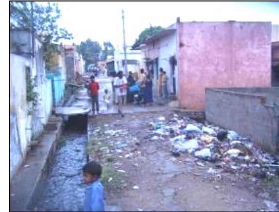
DRAIN NO: BP155 Ch. – 50m. LOCATION: Srinivasapura, near Kogilu Sewage flow in drain is occupying major portion of area Covered drain reaching, providing less scope
